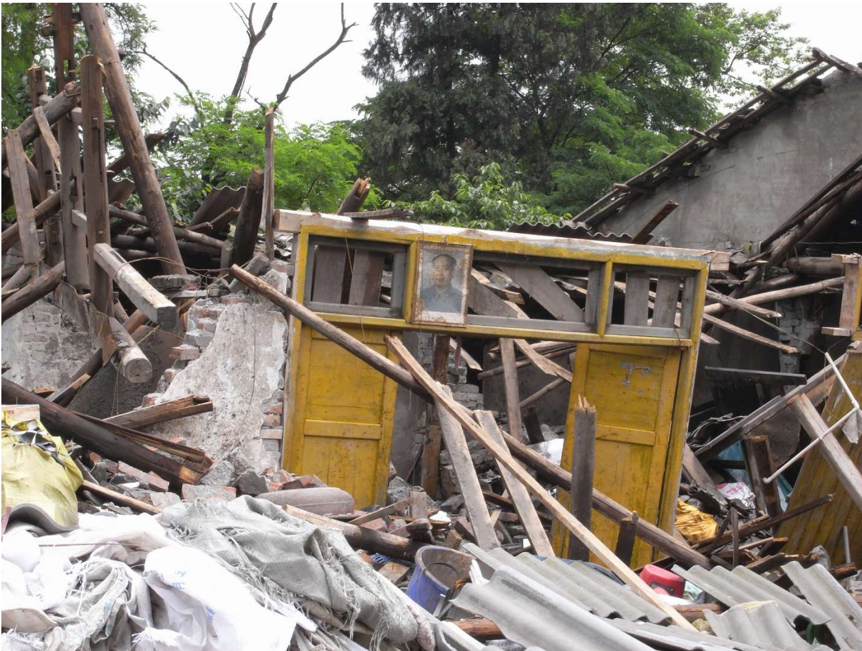
Damage caused by the 2008 Sichuan earthquake on the road heading to Wenyuan, the quake's epicenter, taken on May 14, 2008. Image credit: Miniwiki / Public Domain
